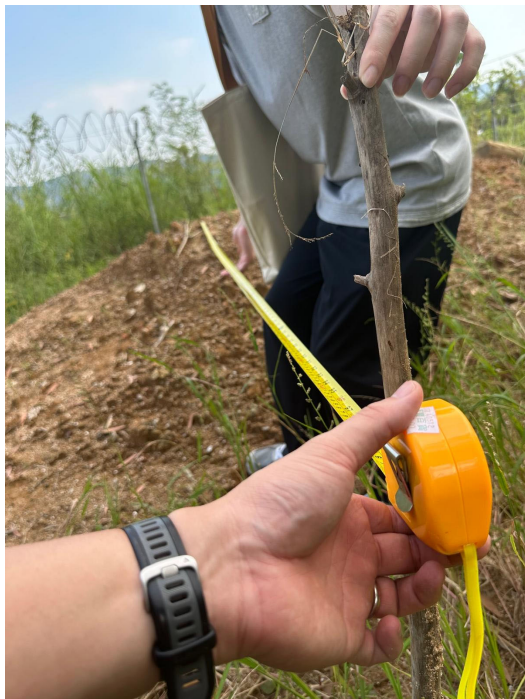
PHOTO11 Site photo for the soil fill to be removed (app. 4.1m(wide) x8.3m(Length)
