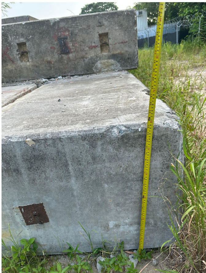
PHOTO 6-8 Site photo for the concrete block type 2 to be removed S.T.WONG & PARTNERS LTD
