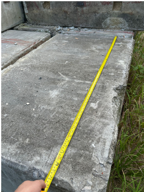
PHOTO 9-10 Site photo for the concrete block type 2 to be removed
